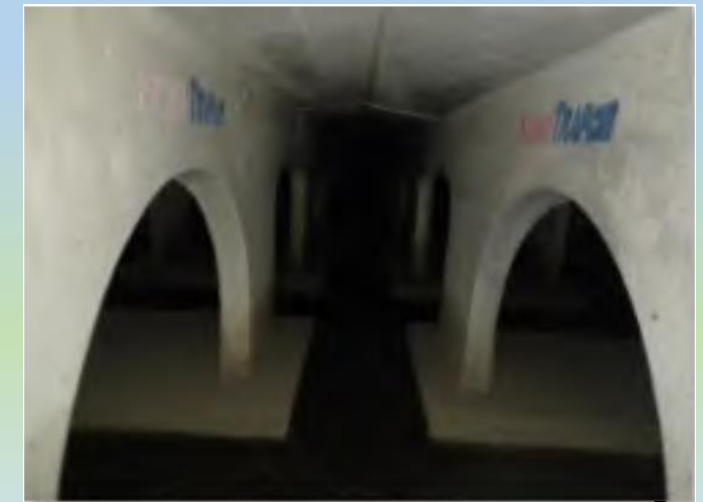
Underground Detention Basin
