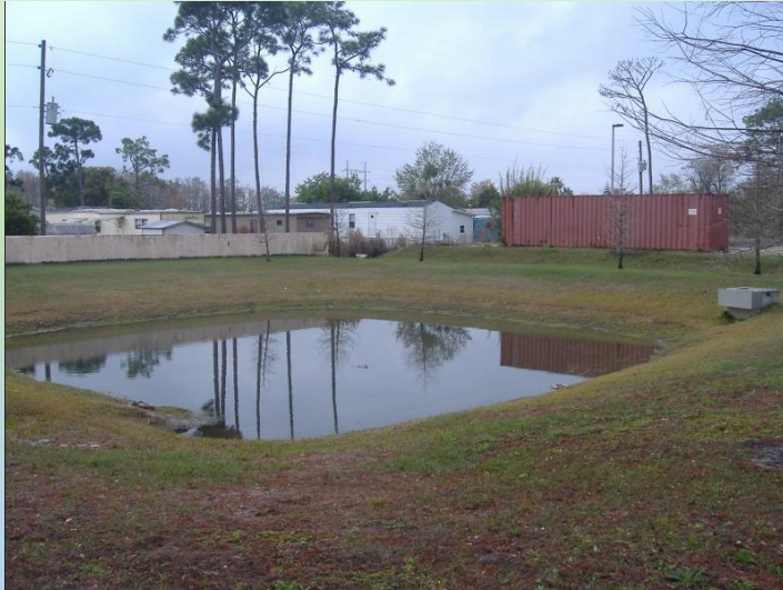
Wet Retention Basin
