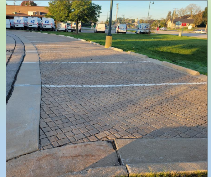
Pervious Pavement / Pavers
