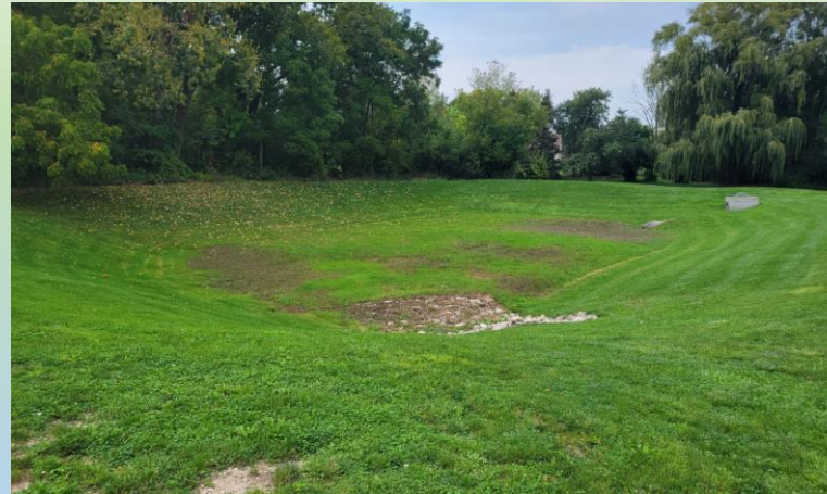
Dry Detention Basin
